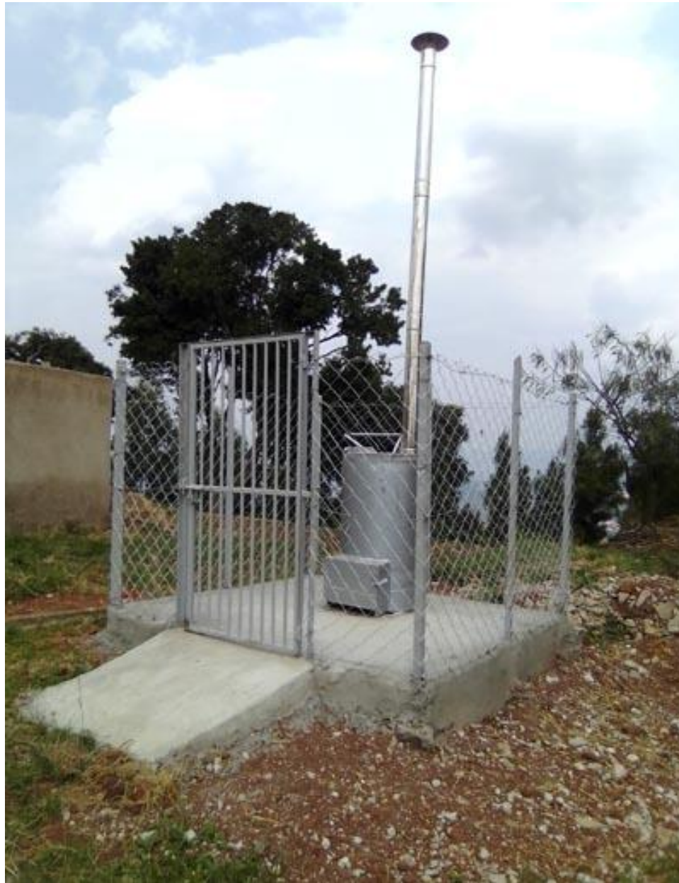
Newly built Incinerator at Rwenzori by WASH – June 2020
